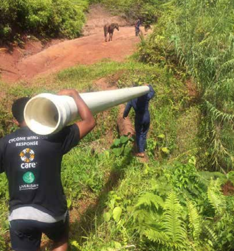
Lifting water pipes across broken logging bridge in Vatuvonu
